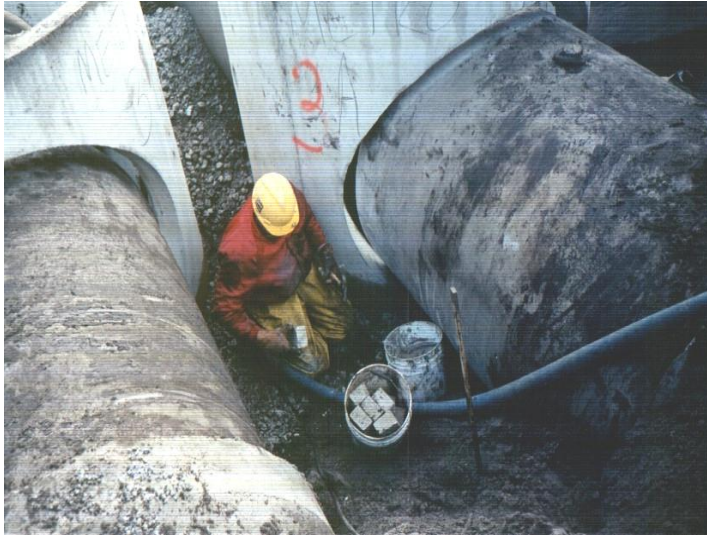
FIGURE 3: Labor Intensive Field Mortaring of Structure Connection
