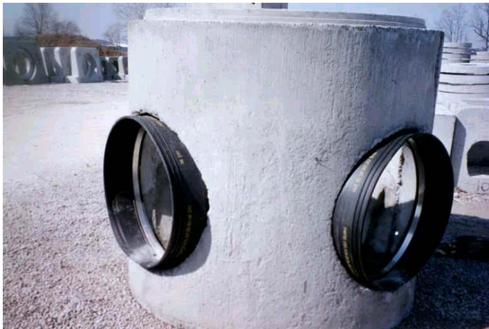
FIGURE 4: Typical Pipe-to-Structure Boot Connection
