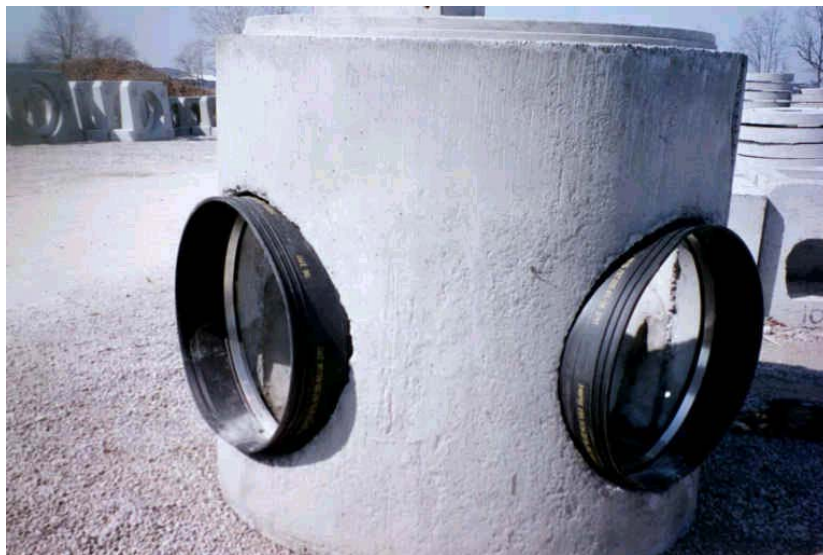
<FIGURE 4: Typical Pipe-to-Structure Boot Connection>
