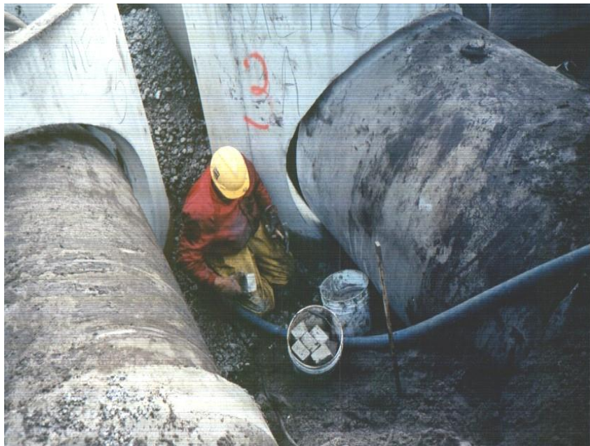
<FIGURE 3: Labor Intensive Field Mortaring of Structure Connection>
