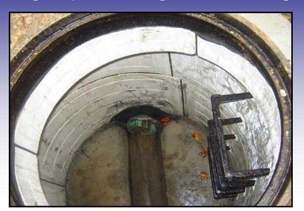
The Dura-Plate lined base with prepoured flow channels was set and connected to the existing clay pipe line in about 20 minutes!
