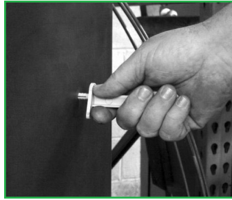
STEP 2: Insert locking mechanism into drilled hole.
