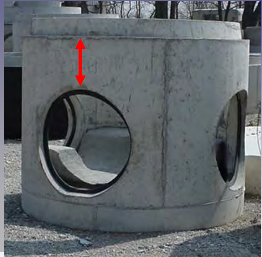
Check the invert elevations by using a common reference point.
