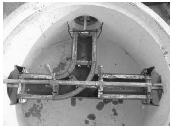
#6 COMPLETED THREE-WAY ASSEMBLY READY TO POUR
